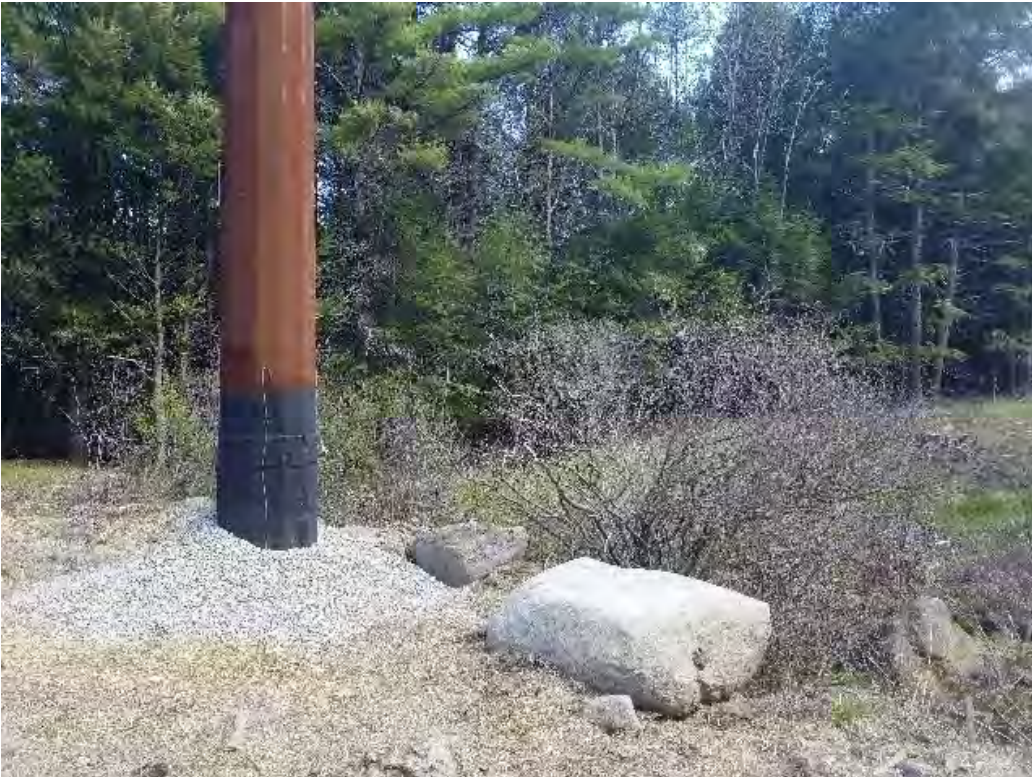
Fig 12: Str. 70 foundation. Viewing north. (05-12-20).
