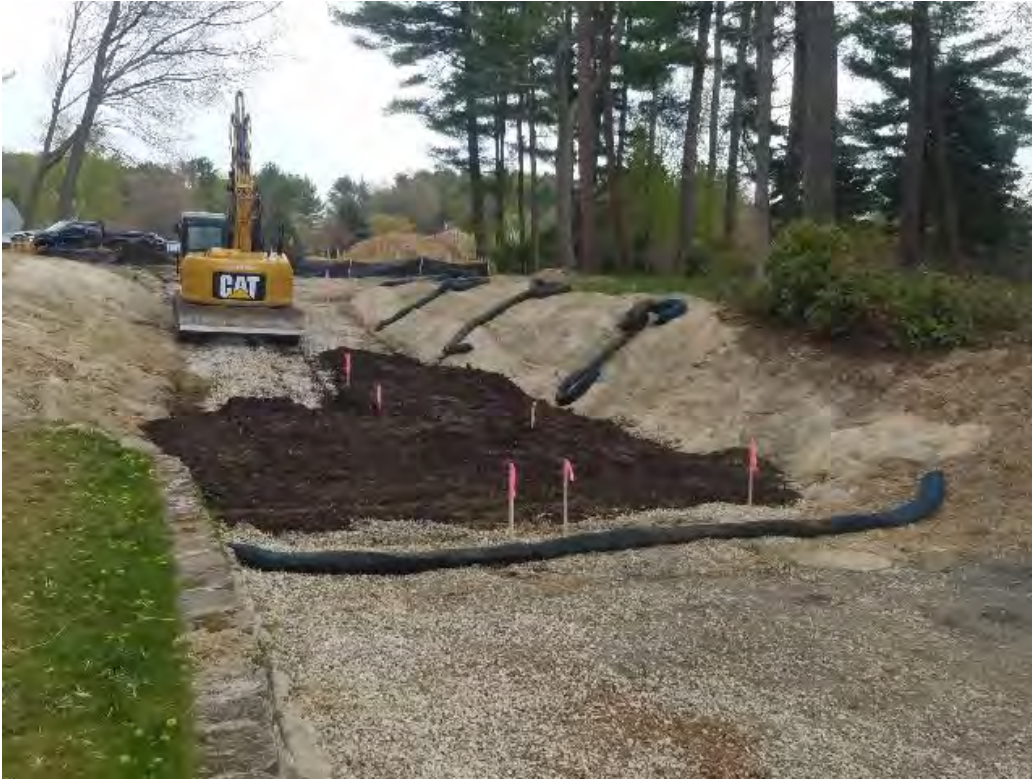
Fig 11: Rye Beach landscaping spreading loam from the manhole up at Gundalow landing/east side of the Bay. Viewing east. (05-11-20).
