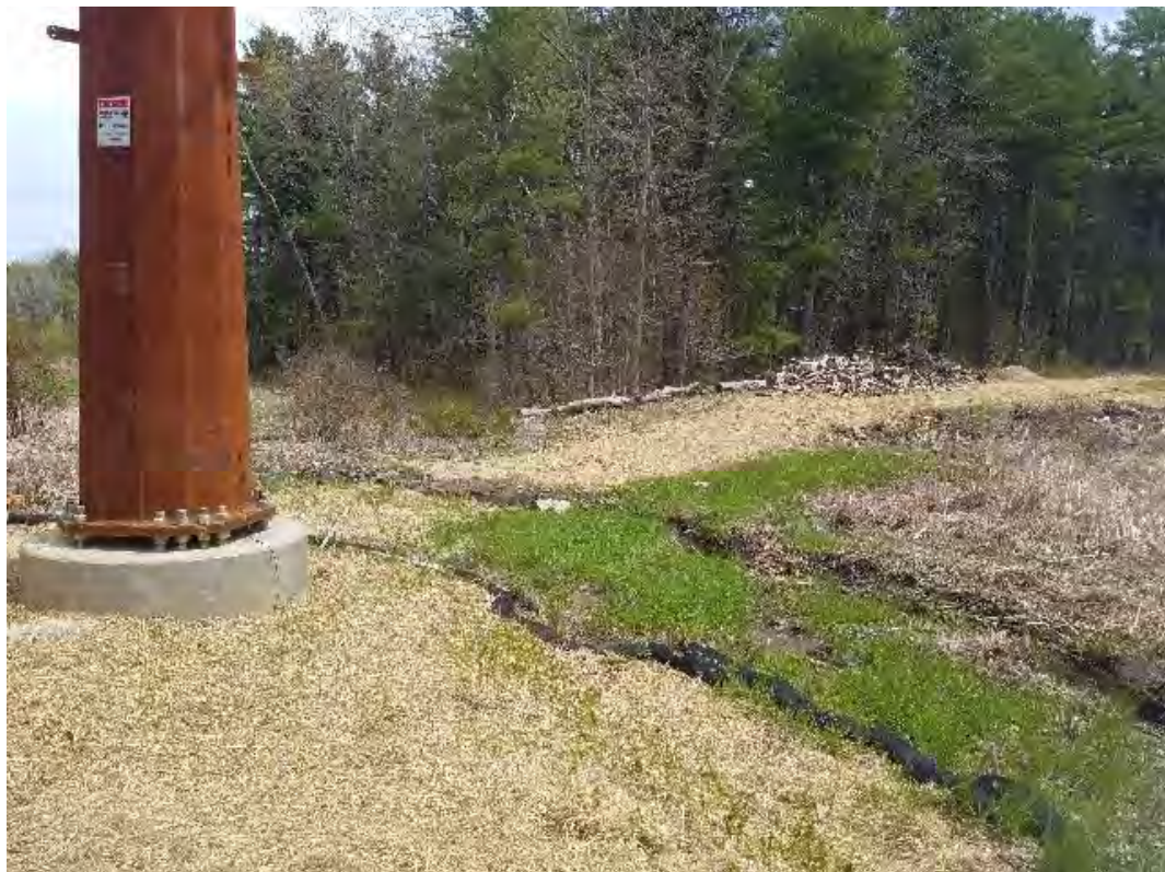
Fig 10: Str. 112 foundation next to wetland NW34. Viewing northeast. (05-11-20).
