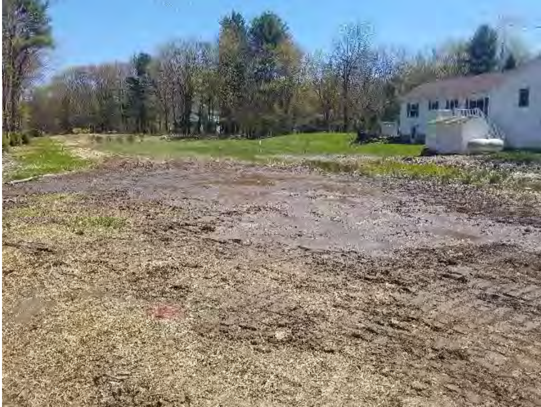
Fig 17: Wetland NW22 restoration in progress. Viewing east. (05-13-20).
