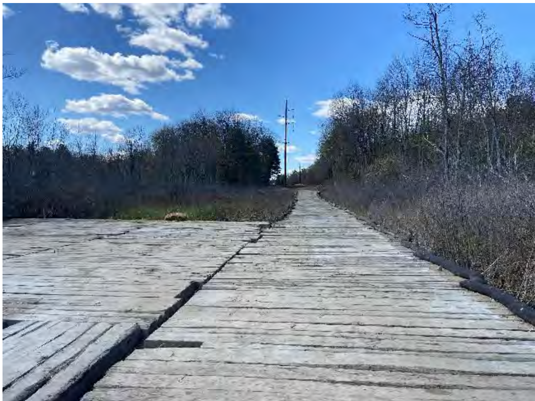
Fig 2: Access road to Str. 35, though wetland DW41. Viewing southwest. (05-07-20).
