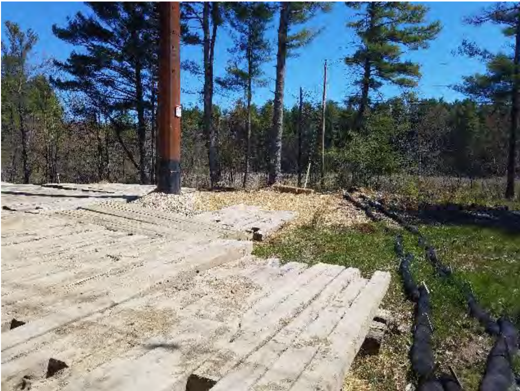
Fig 14: Str. 94 pole and work area. Viewing north. (05-13-20).
