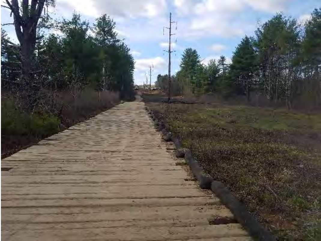
Fig 5: Access road between Strs 43-44, adjacent to wetland DW58. Viewing south. (05-08-20).
