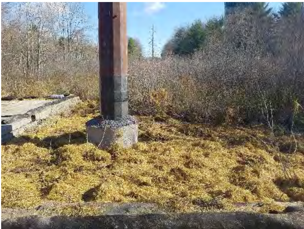
Fig 6: Str. 35 foundation. Viewing north. (05-08-20).
