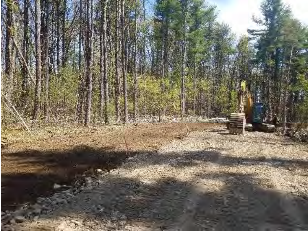
Fig 9: Progress of the relocation of the access road at Flynn Pit. (05-11-20).
