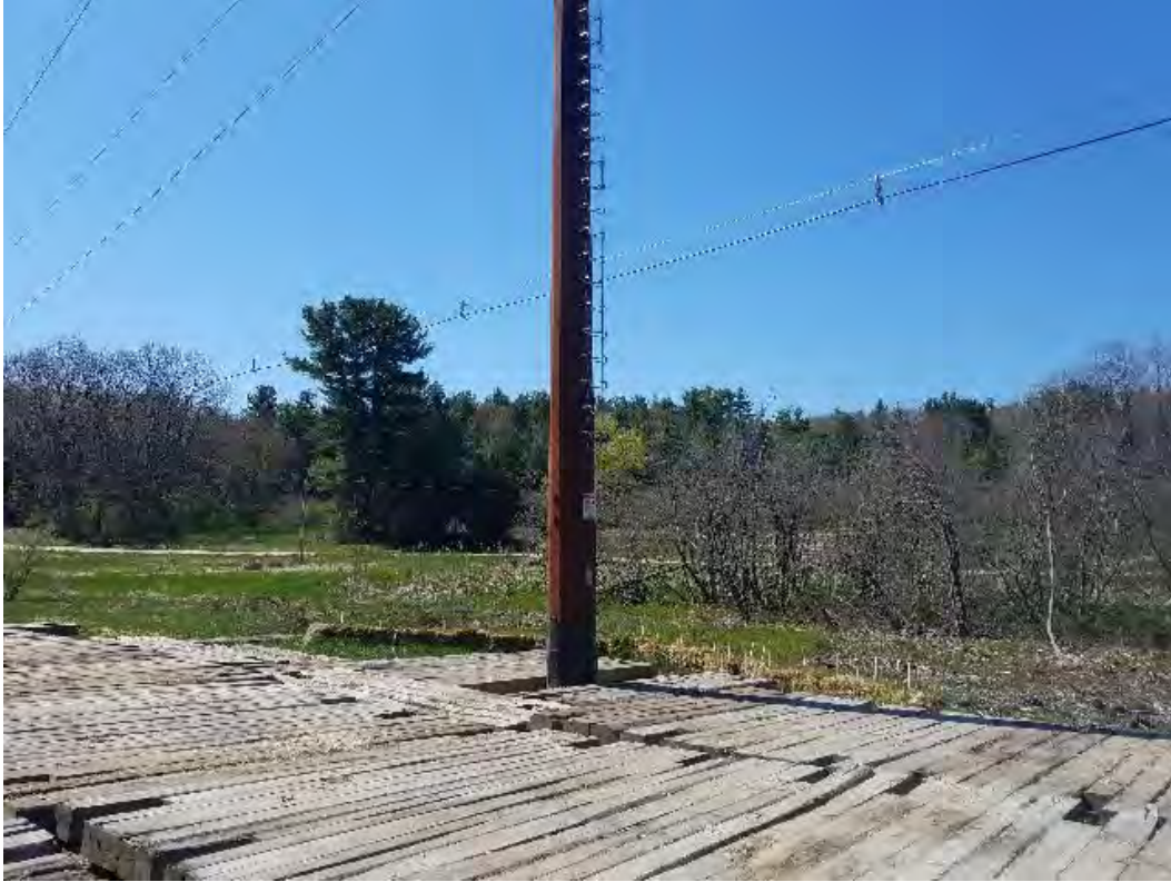
Fig 15: Str. 95 pole and work area. Viewing south. (05-13-20).
